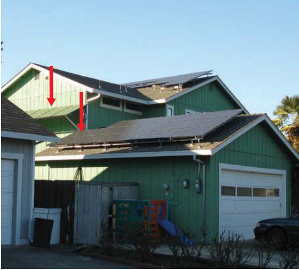
Figure 1. 6.4 kW Installation: Arrows show shade locations
