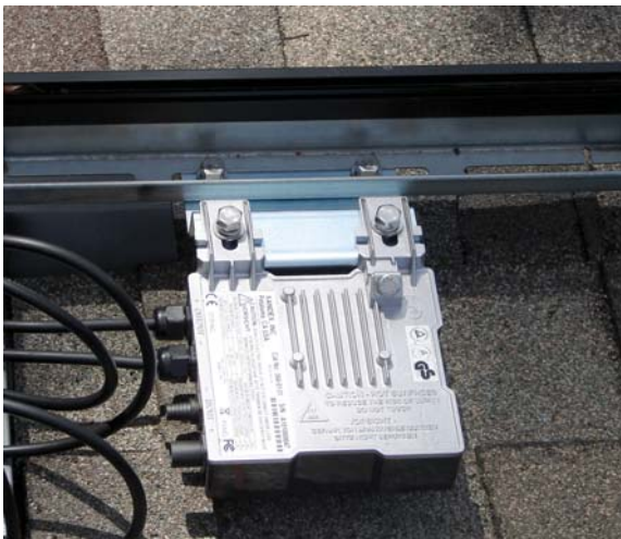
Figure 3: SunMizer units installed under module locations
